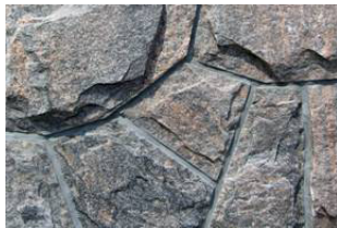
Stone Material for Decorative Masonry Features (Split-face Muskoka Granite)
