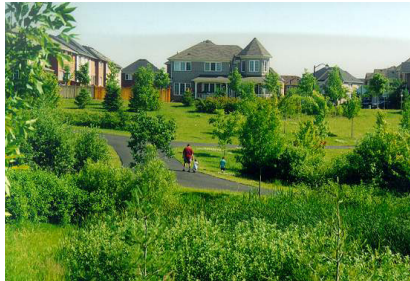
Figure 1.3b - Stormwater Management Facility
